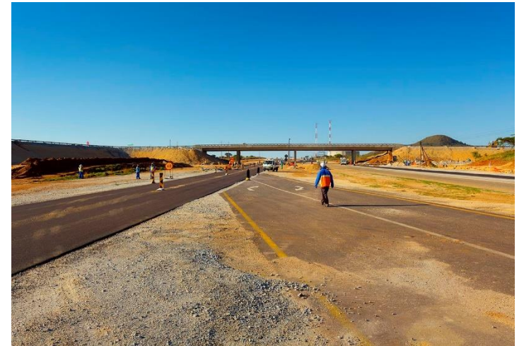
R37 Provincial road upgrades around Polokwane smelter
